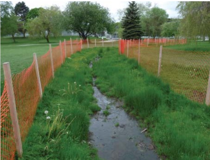
Figure 3.8: Rainwater bioswale garden
