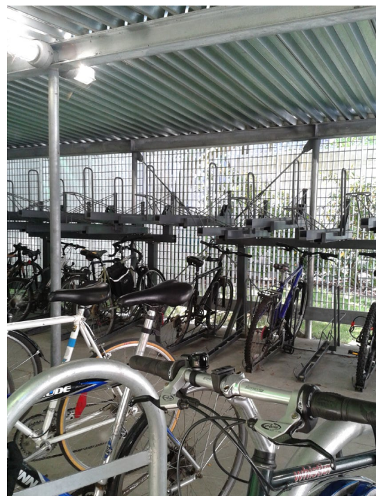
Example of a facility combining the simple bike racks (in front), and double deck racks.
