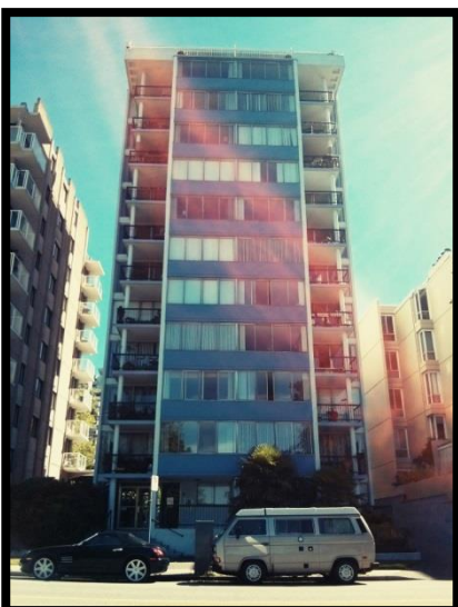
Beach Ave Pilot Building
