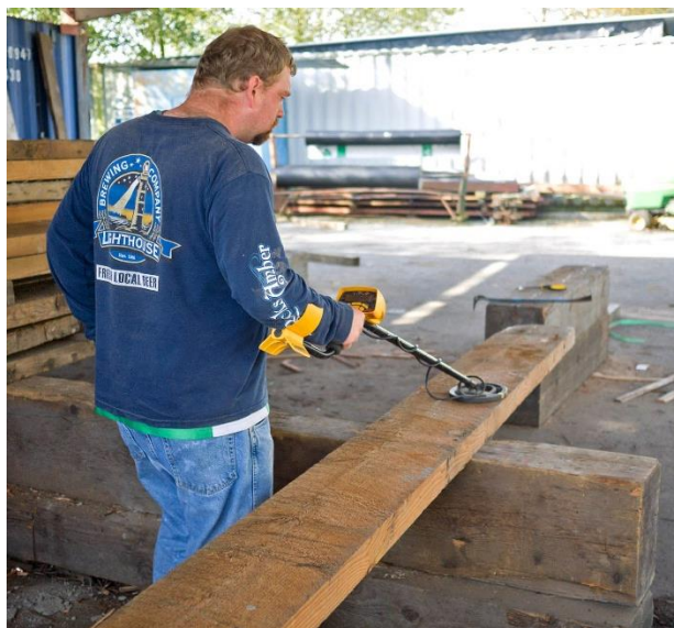
Figure 10 Using metal detector to ensure there is no metal in the wood for re-milling (West Coast Reclaimed Lumber)
