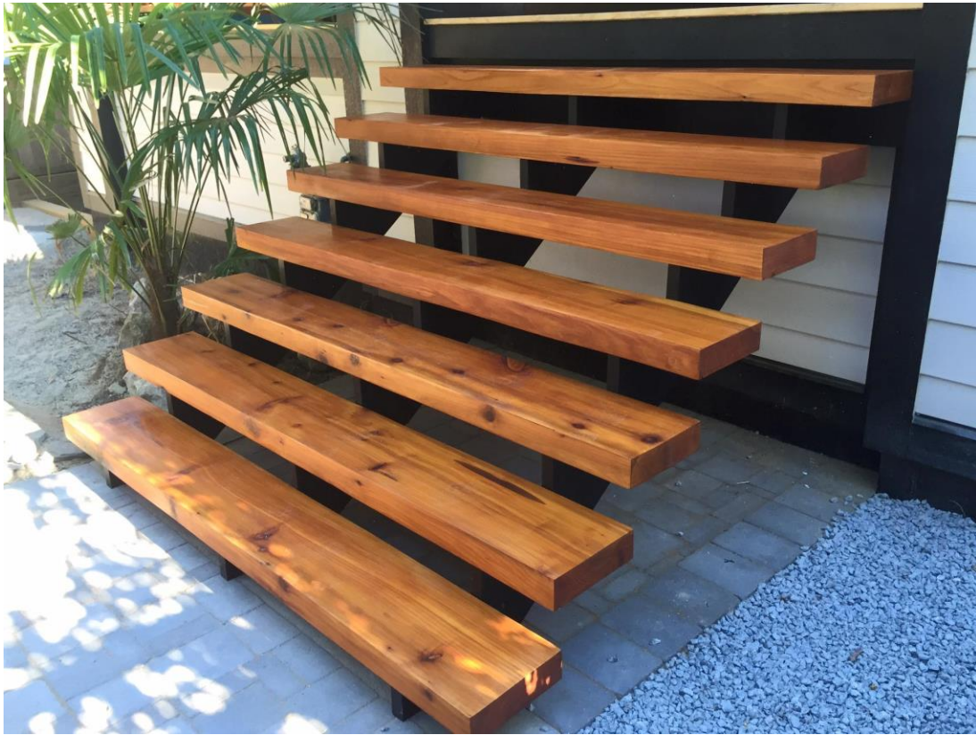
Figure 32 Stair case ( Naturally Crafted Construction )
