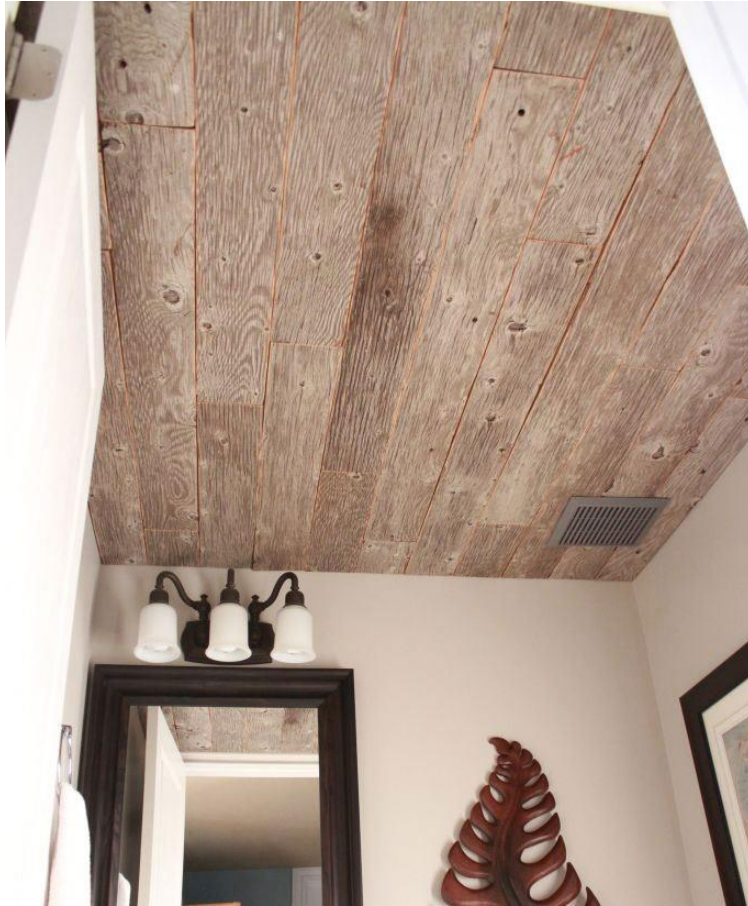
Figure 15 Reclaimed board used in ceiling
