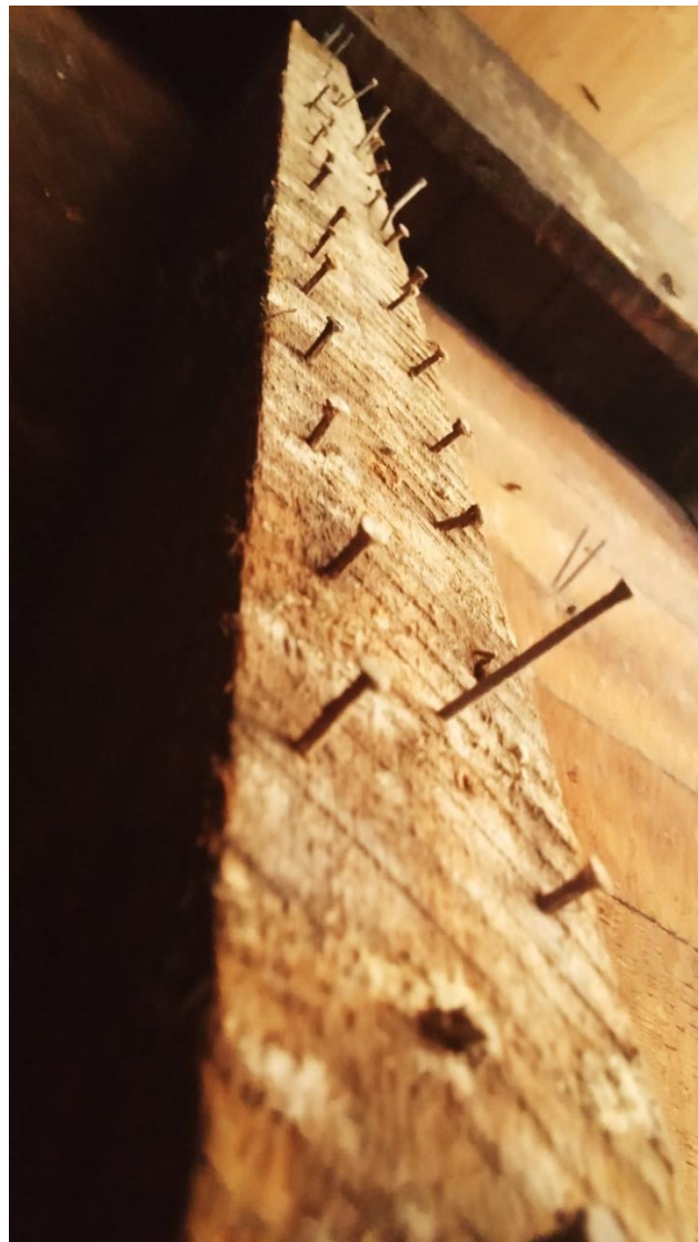
Figure 6 Some dimensional lumbars (specially 2×4 wall studs) have lots of nails which require a lot of labour to remove
