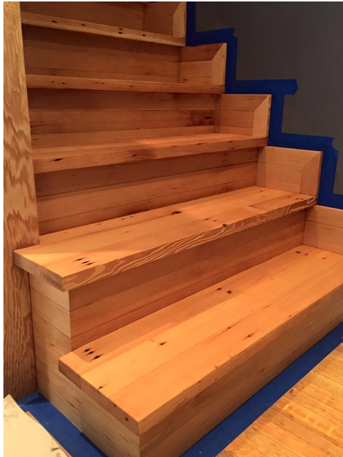
Figure 19 Stair treads built from salvaged 2x4 lumber ( Naturally Crafted Construction )
