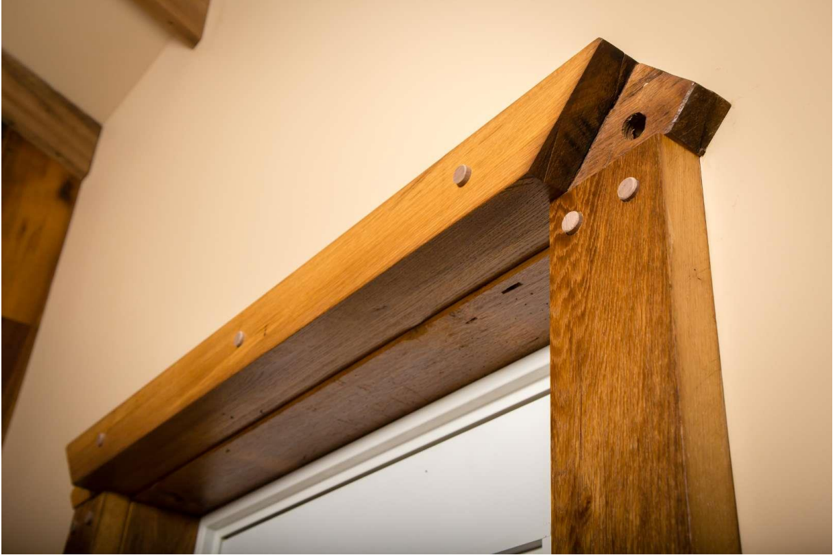
Figure 22 Window trim from salvaged wood ( Pure Nard Woodworking )
