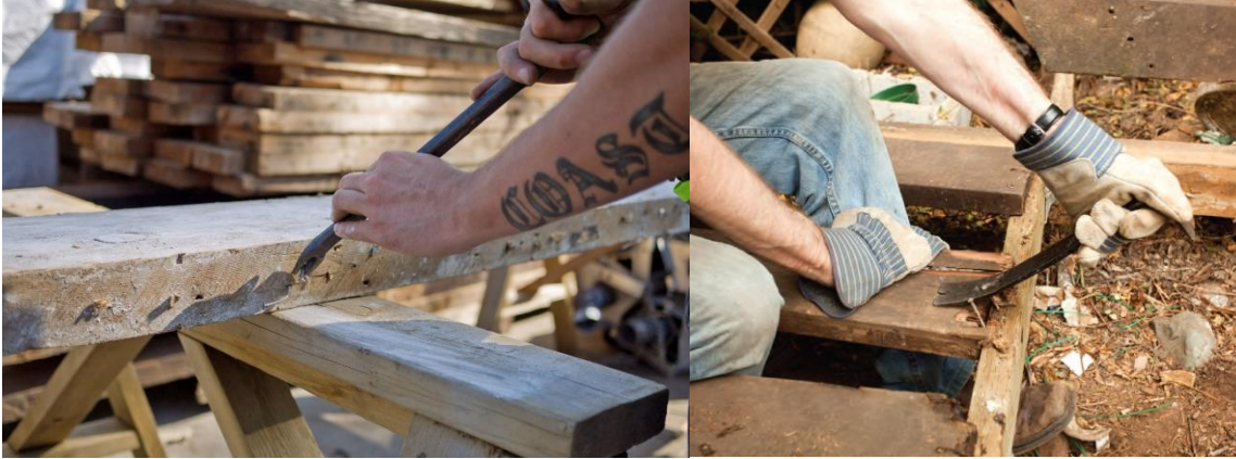
Figure 8 De-nailing of lumber (the source for the picture on the right: (Delta Institute, 2012))
