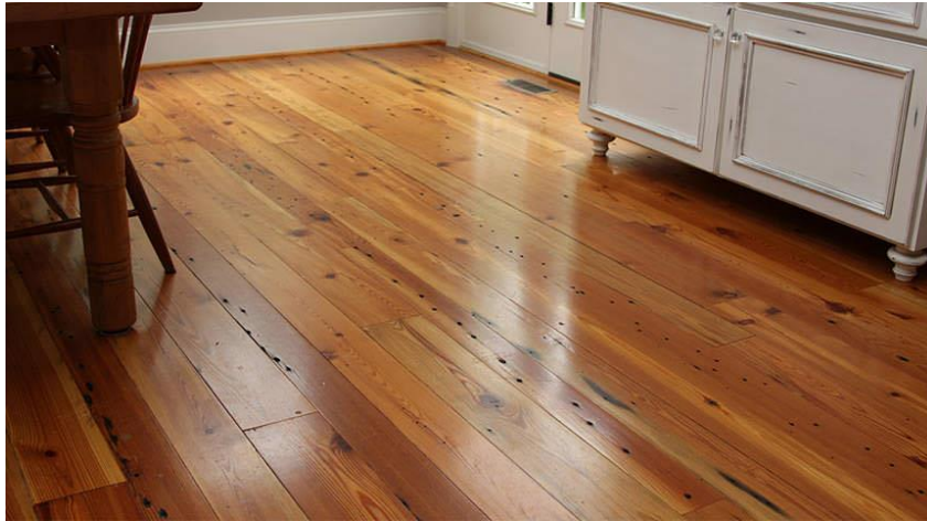
Figure 13 Kitchen Floor Made With reclaimed wood with nail holes on it ( E.T. Moore Manufacturing )
