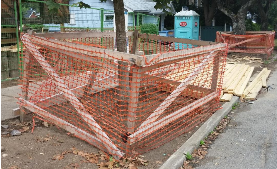
Figure 38 Temporary tree protection during construction
