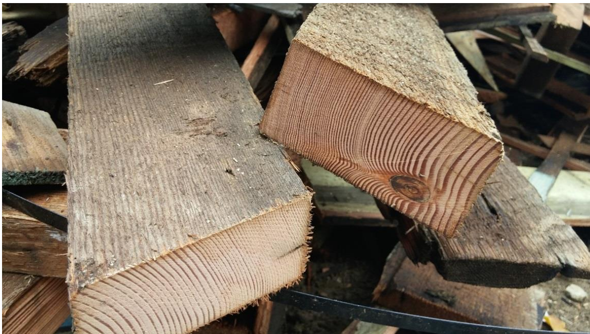
Figure 3 A section view of a 2x4 lumber taken out from a 1920s heritage house in Vancouver (735 22nd e)
