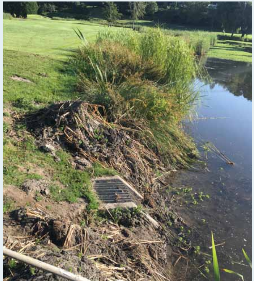
The pump at left is a stopgap solution to prevent flooding while waiting for a debris blasting service. The drain at right is not protected and requires daily clearing of debris to prevent clogging. photo credit: Jennifer Rae Pierce
