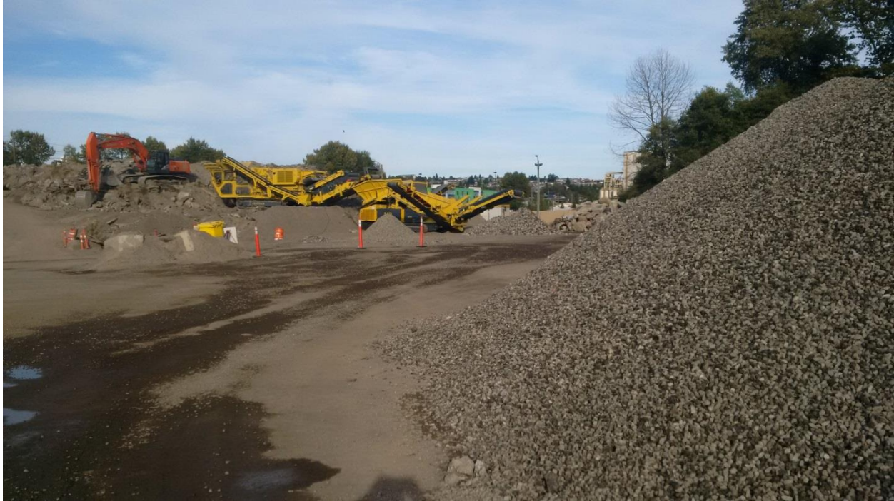
Figure 2: Kent Yard recycled aggregate production (Photo Courtesy of Kent Yard)
