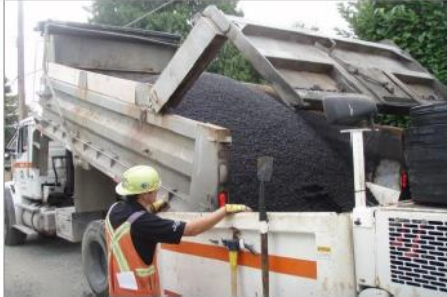
Warm mix asphalt with 20% recycled content
