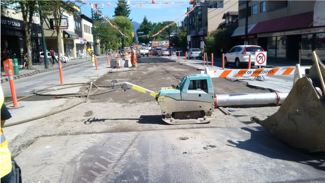
Recycled aggregate used as trench fill
