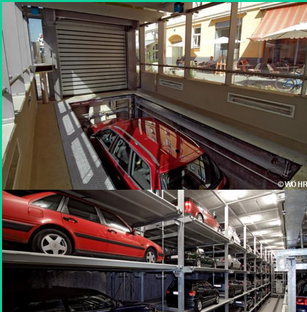
Figure 11: A transfer station and underground parking storage for Munich's automated parking.
