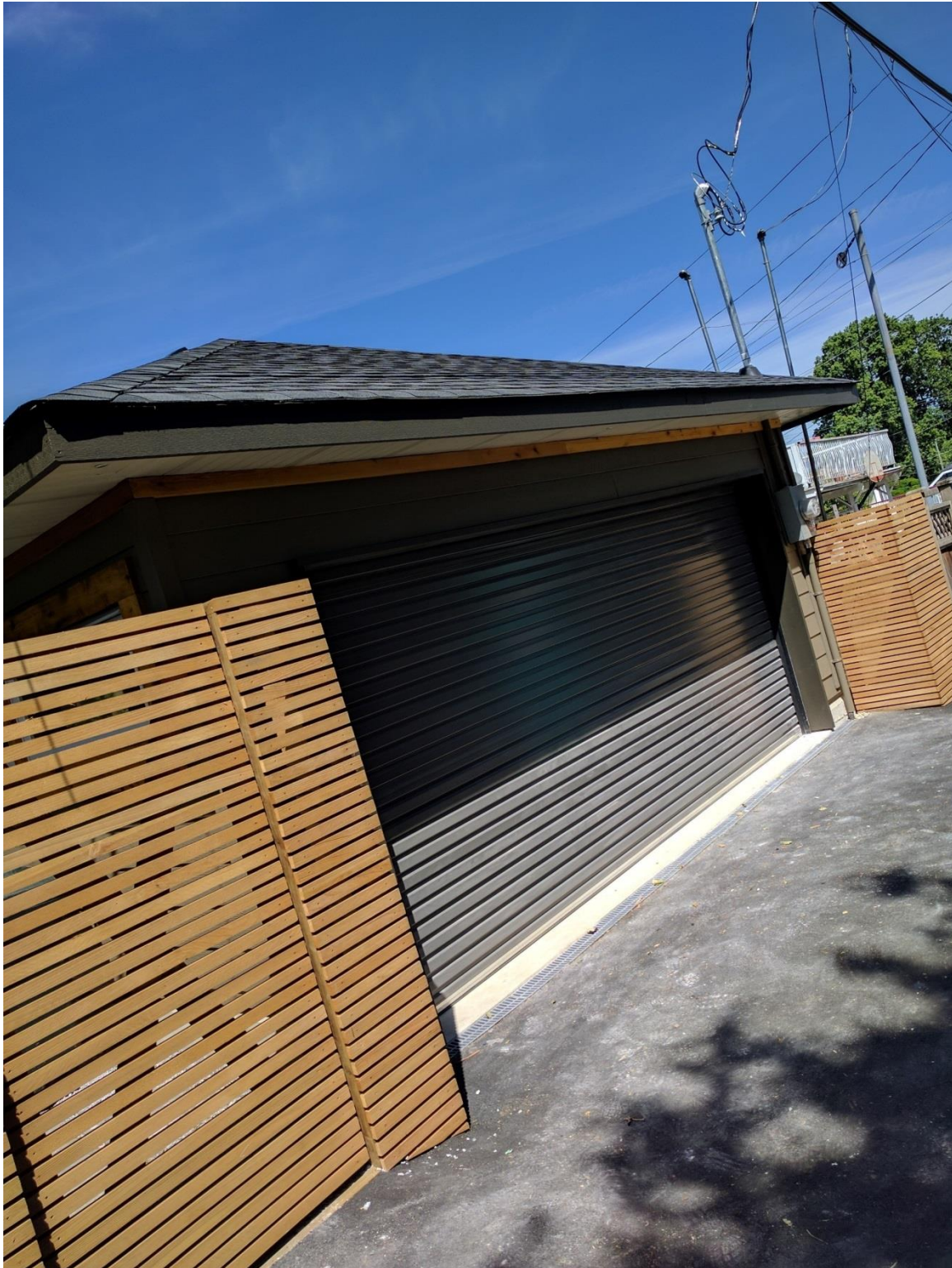
Photo 3: A view of the new parking garage.
