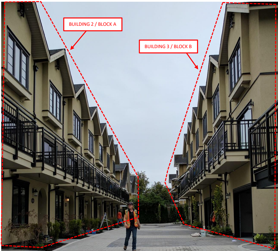
Photo 3: A view of the residential multifamily building located at 4330 Knight Street.
