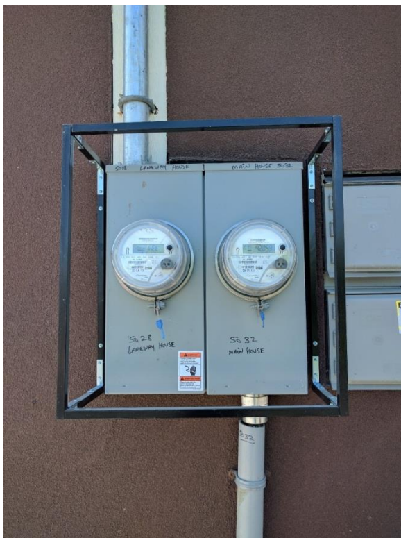
Photos 1 and 2 (L-R): An external view of the LV metering for the incoming electrical supply at the Laneway House; an internal view of the new electrical panel located at the on-grade, open-to-sky parking area.
