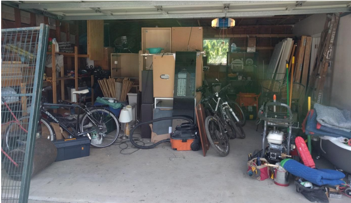
Photo 3: A view of the existing garage, which was adapted to accommodate the new Electric Panel, seen in Photo 2.
