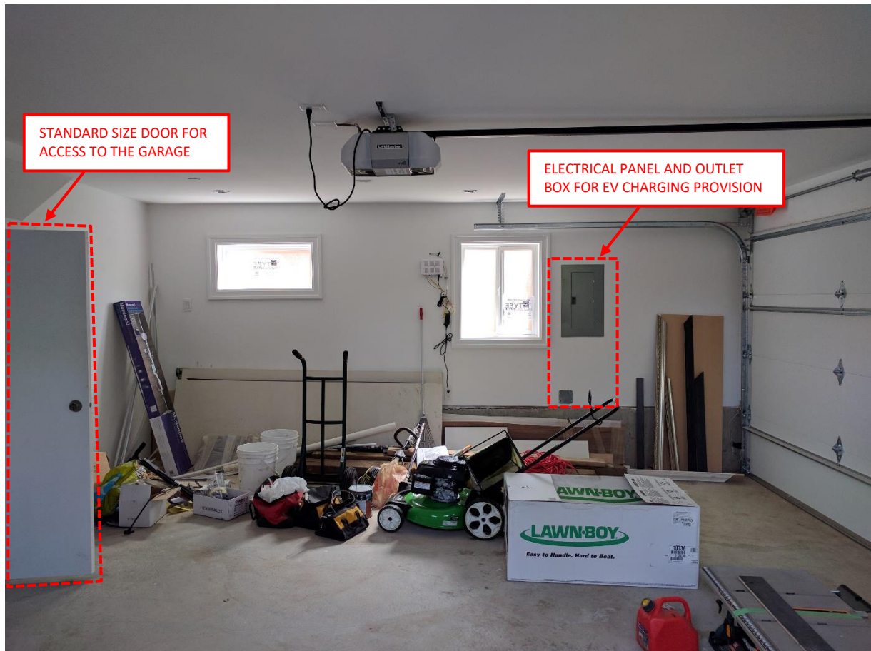
Photo 5: A view of the built-in two-car garage at the Laneway House.
