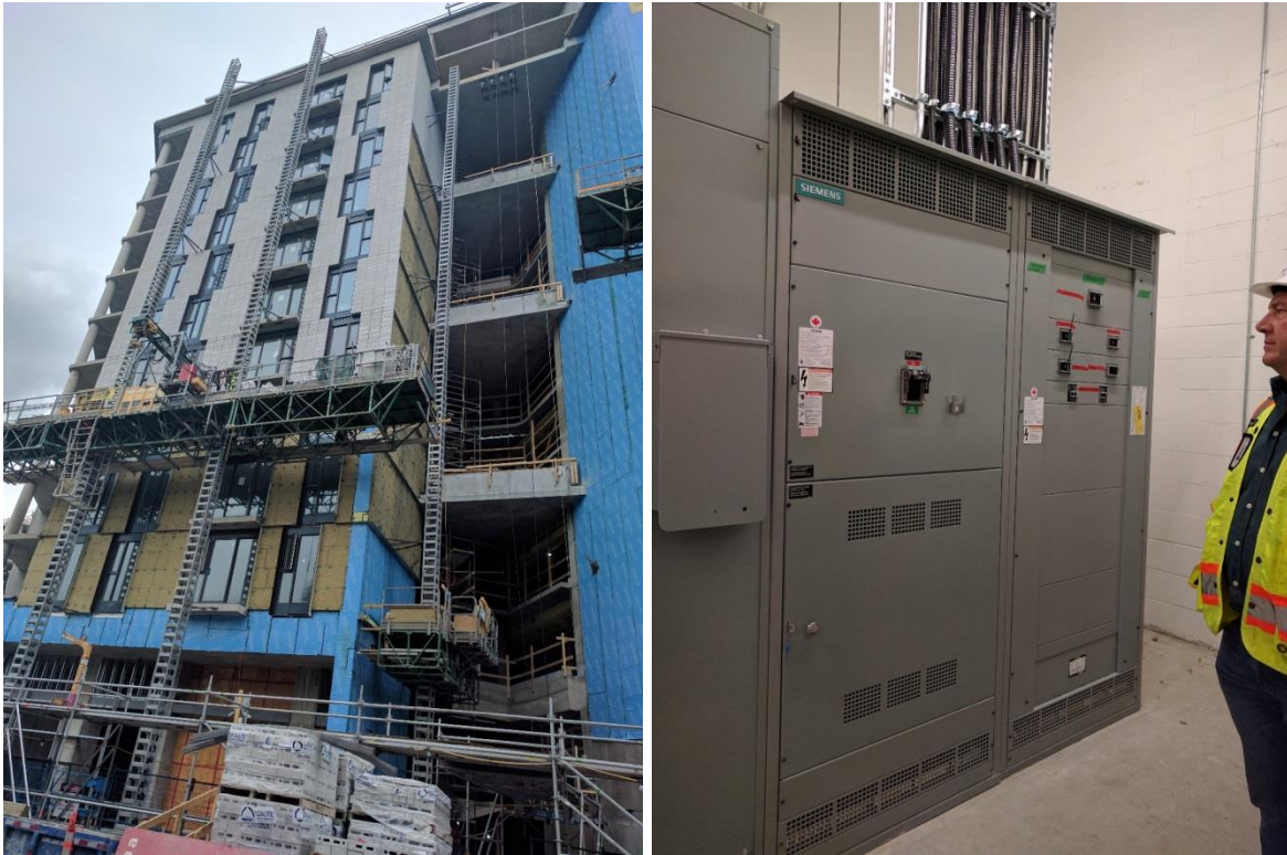
Photos 2 and 3 (L-R): A view of the mixed-use building located at 333 East 11th Avenue; A view of the step-down electrical switchgear located at the electrical room.
