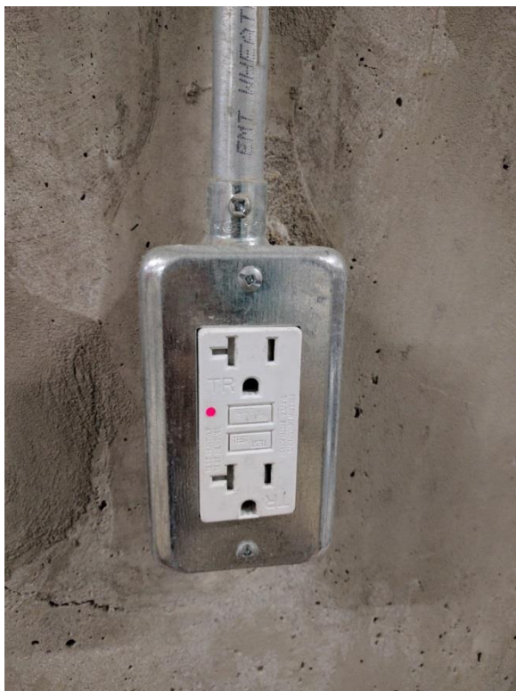
Photos 8 and 9 (L-R): A close-up view of the dedicated EV charging receptacle, capable of supplying 120-V / 20-A, mounted on the walls of the underground parkade; A close-up view of the Electrical Single Line Diagram, wherein the highlighted region shows the pertinent note necessitating EV charging receptacles.
