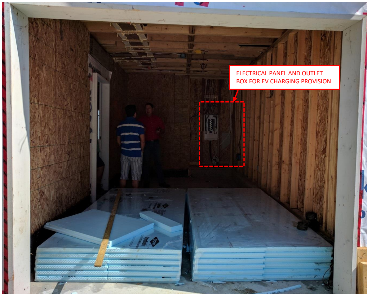
Photo 4: A view of the attached parking garage providing one parking space with vehicle access from the lane.
