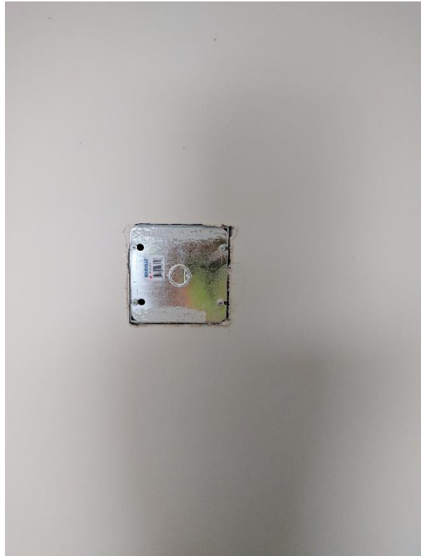
Photos 4 and 5 (L-R): An internal view of the local electrical panel, located at the parking stall, supplying a dedicated outgoing branch circuit capable of supplying 240-V / 40-A to the EV charging outlet box; A close-up view of the outlet box mounted on the wall.
