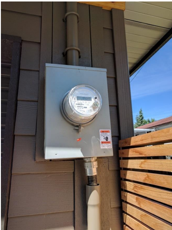
Photos 1 and 2 (L-R): An external view of the LV metering for the incoming electrical supply at the One-family Dwelling; An internal view of the new electrical panel located at the parking garage.
