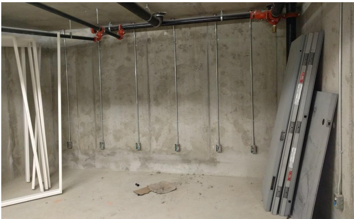
Photos 6 and 7 (T-B): A view of the car parking section of the underground parkade, where 20% of the parking stalls are provided with dedicated 240-V / 40-A EV charging receptacles; A view of the bike parking section of the underground parkade, where 100% of the parking stalls are provided with dedicated 120-V / 20-A EV charging receptacles;
