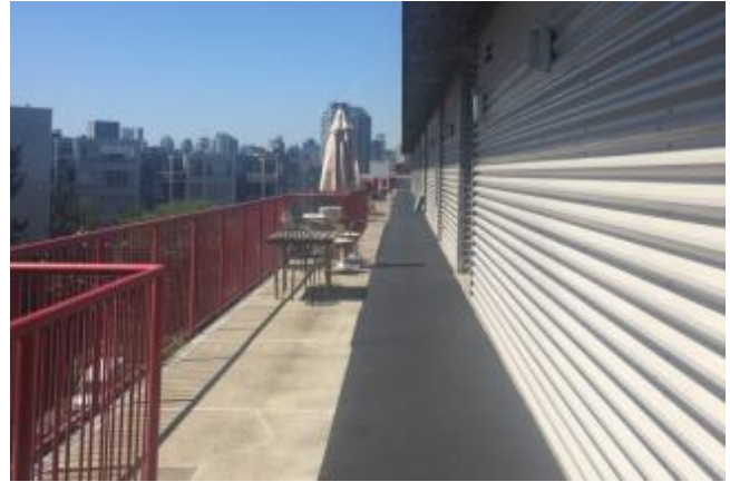
Corridors at Mainspace
