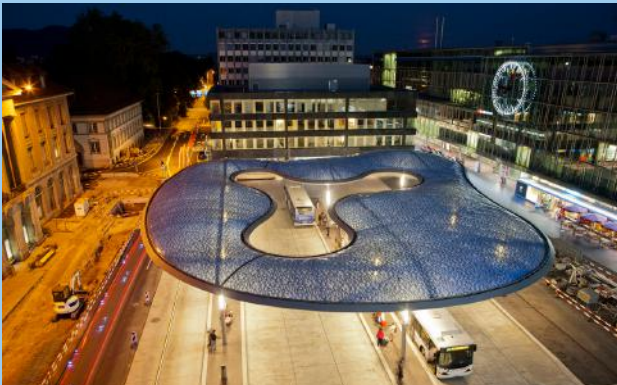
Aarau bus station canopy (Niklaus Spoerri/ArchDaily)
