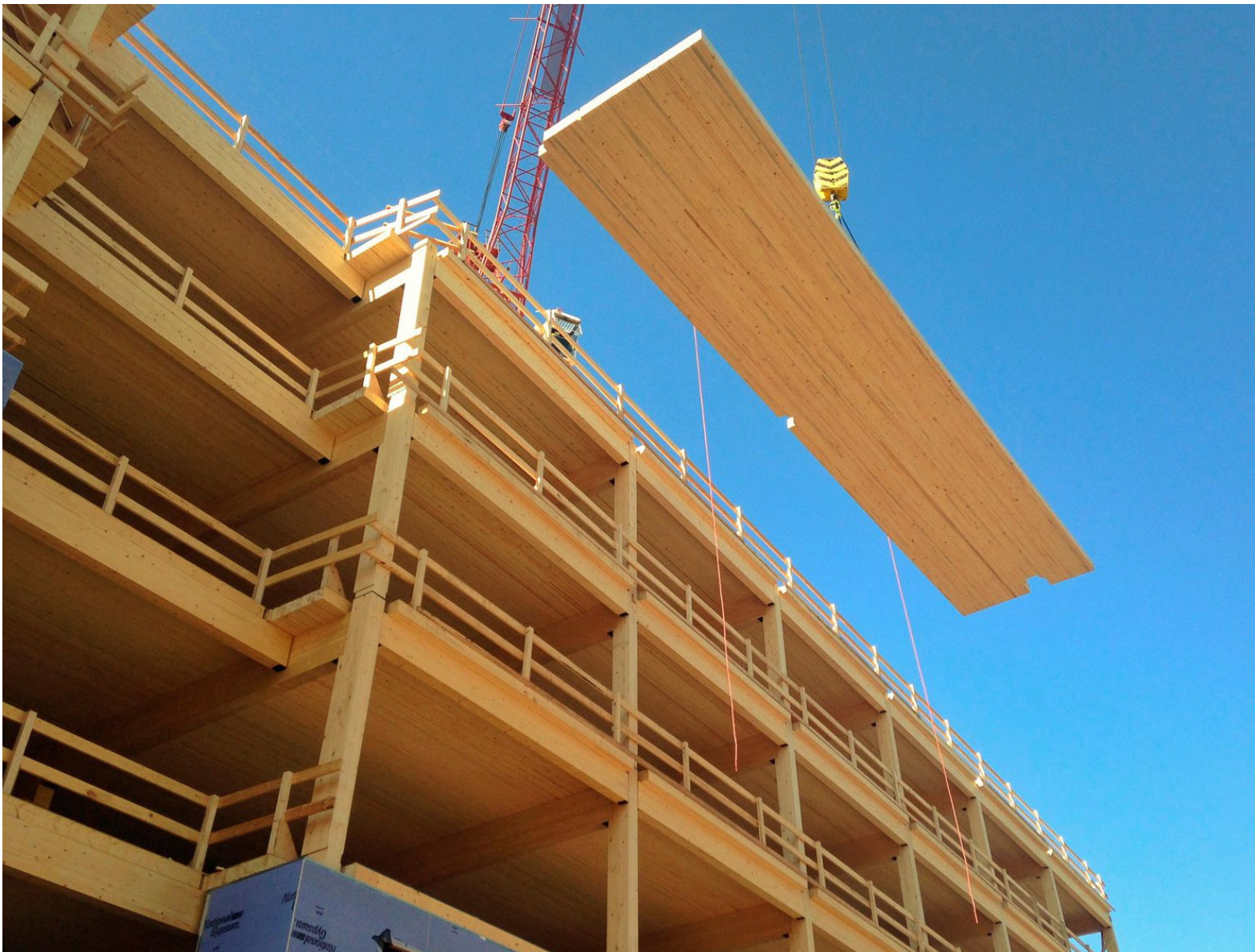
Generally, wooden construction is considered to have a lower embodied carbon than a comparable sized concrete building. Image by Jimmy Stamp via Smithsonian magazine .
