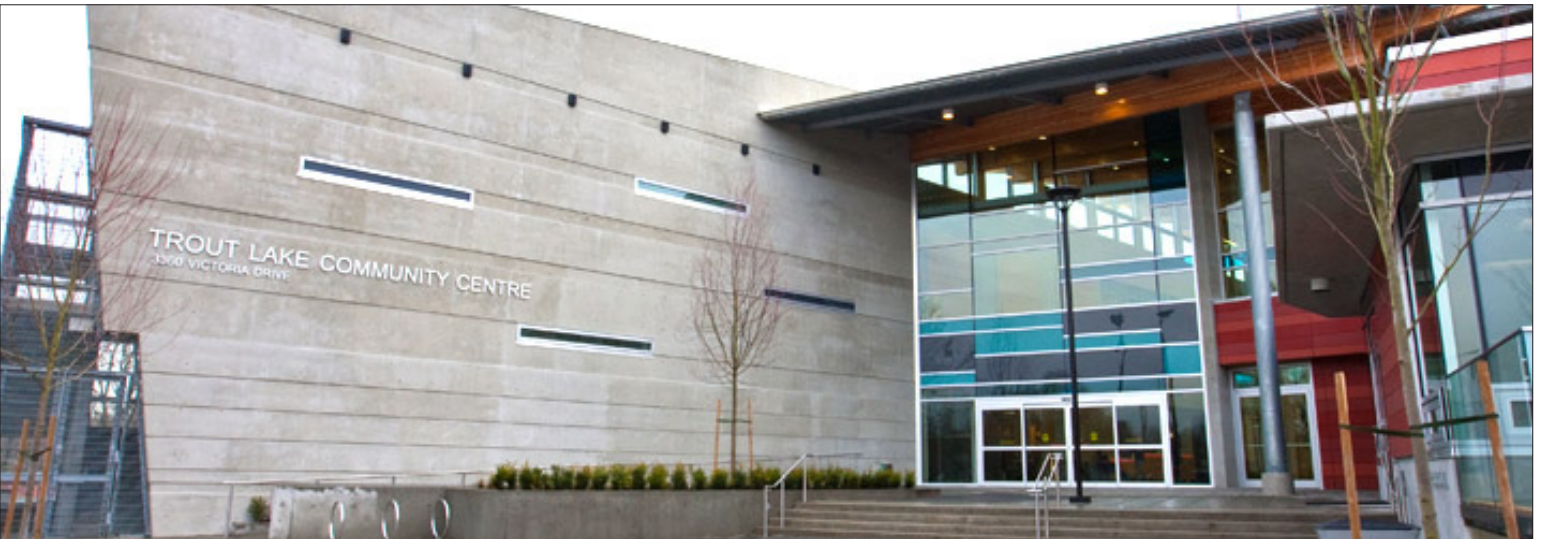
Public facilities such as libraries and community centres are an integral component of a healthy and resilient neighbourhood. Photo of Trout Lake Community Centre (Vancouver) sourced from the City of Vancouver .
