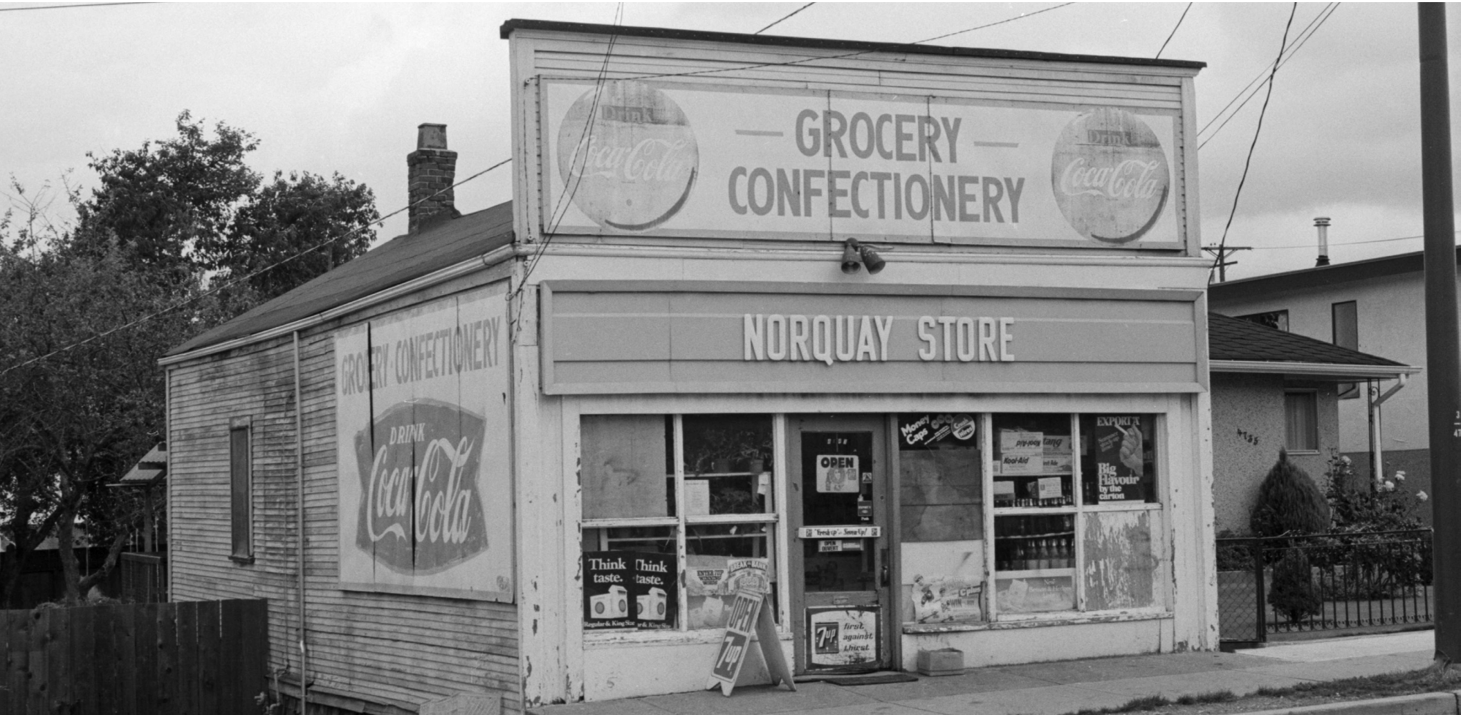
Norquay Store at 4743 Slocan St (1978); City of Vancouver Archives.
