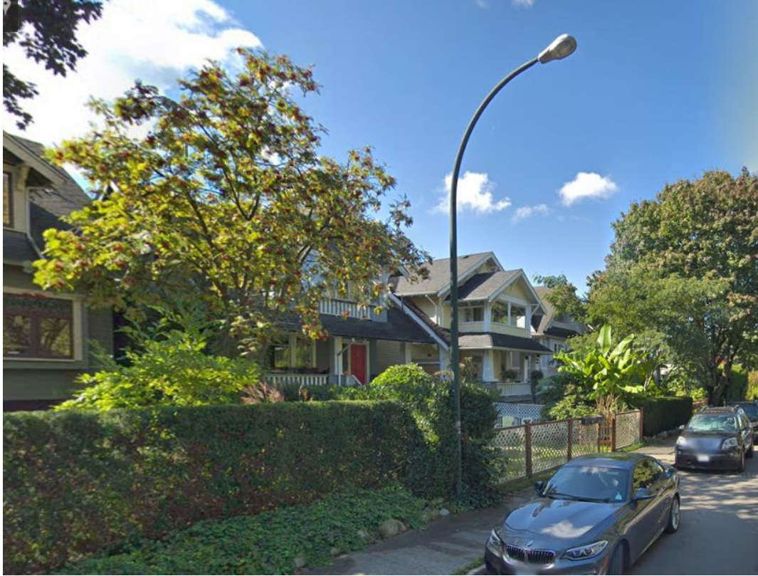
Figure 13. Light pole on the wrong side of the sidewalk.
