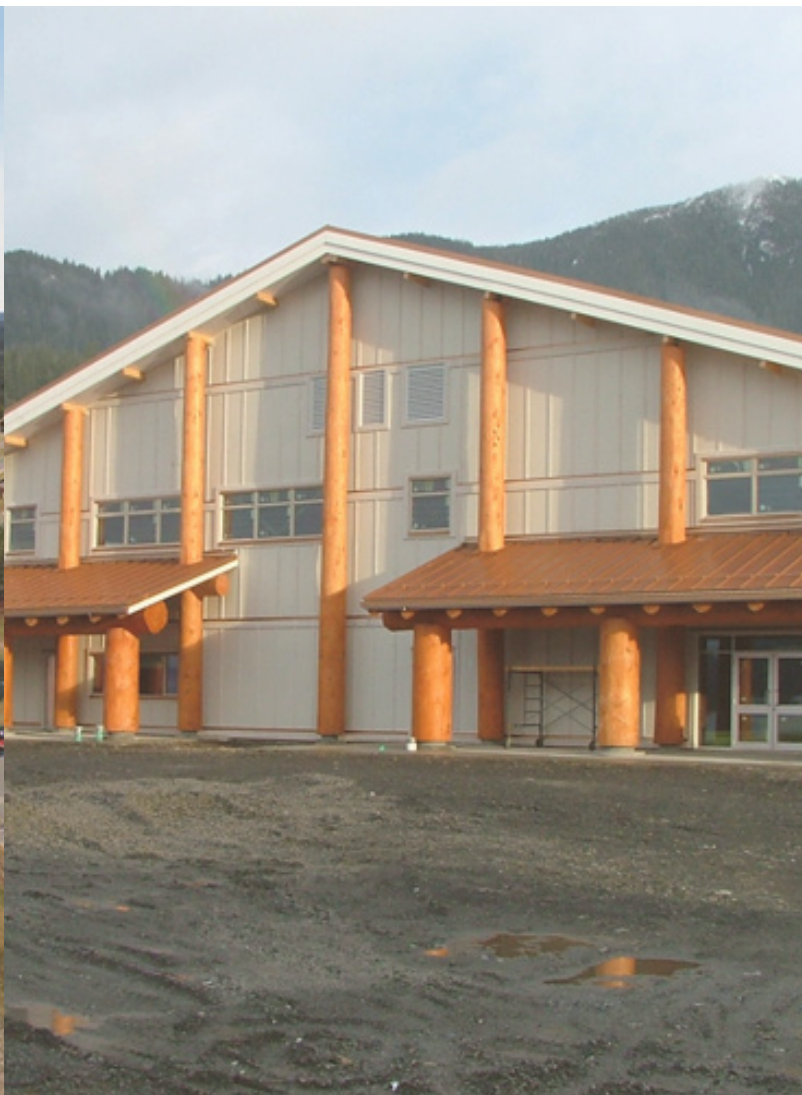
Gingolx Community Hall Photo credit: Patrick Stewart Architect
