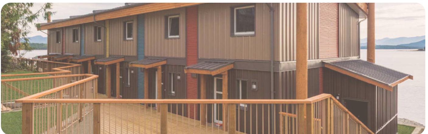
Multi-unit Passive House, Heiltsuk First Nation. Photo credit: Britco LP.
