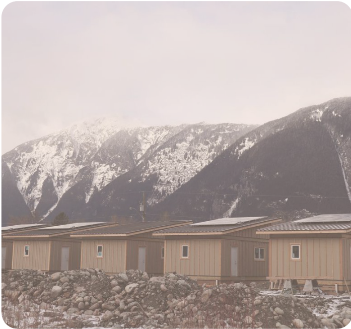
Nuxalk Tiny Homes, built by carpentry apprentices. Photo credit: The Canadian Press
