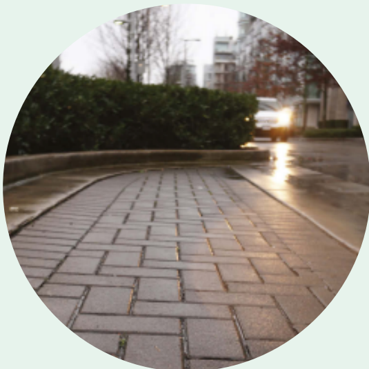
Permeable Pavement in the City of Vancouver. Source: City of Vancouver GRI Typologies.
