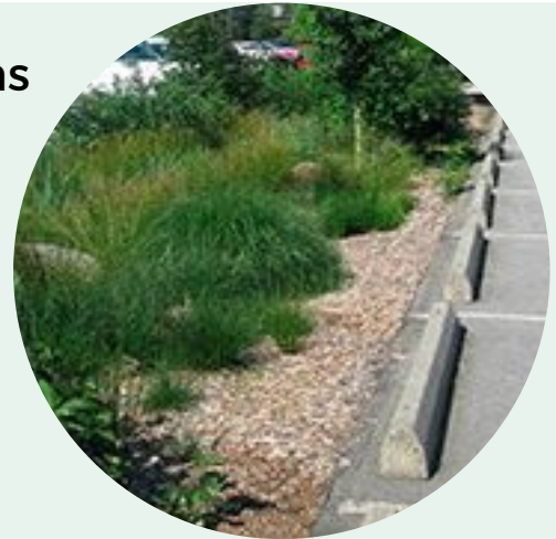
The City of Coquitlam has incorporated Bioswales in parking lots. Source: City of Coquitlam, Featured Projects
