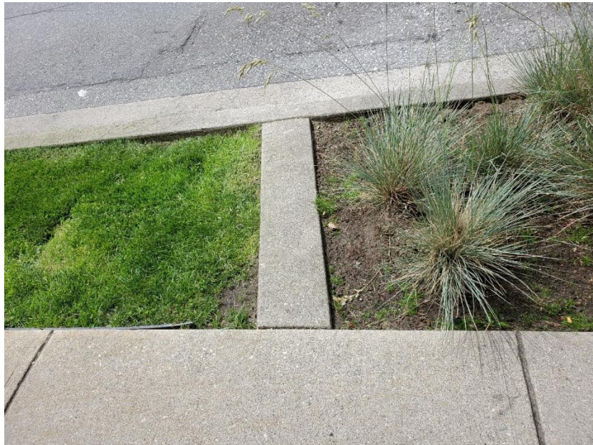
Figure 6: Street side separated bioretention bulges with different vegetation cover, Pine St, Vancouver, BC, 2020.
