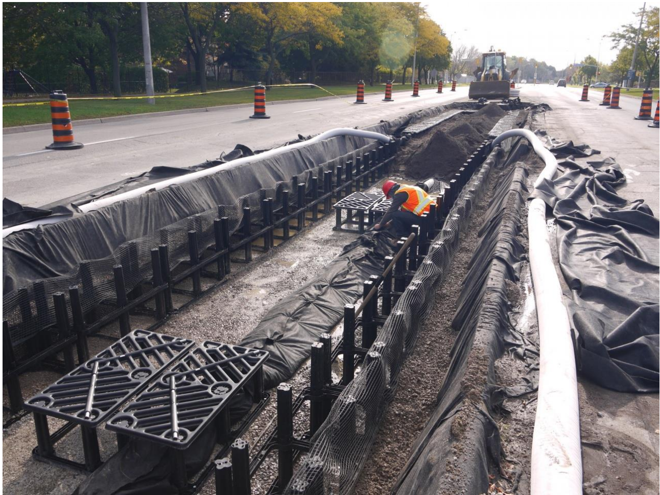
Figure 13: Soil cell installation on Central Parkway in Mississauga
