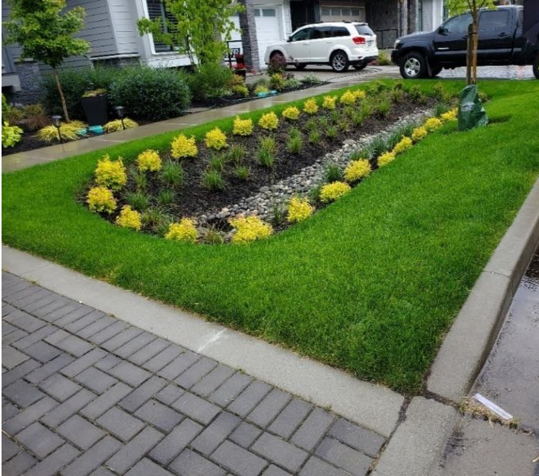
Figure 8: Sunnyside Drainage Corridor Bioswale and Pervious Pavers combined bioretention practice.
