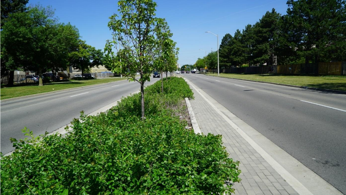
Figure 12: Built in 2014, this stormwater planter on Central Parkway in Mississauga uses supported soil cells and is functioning well.
