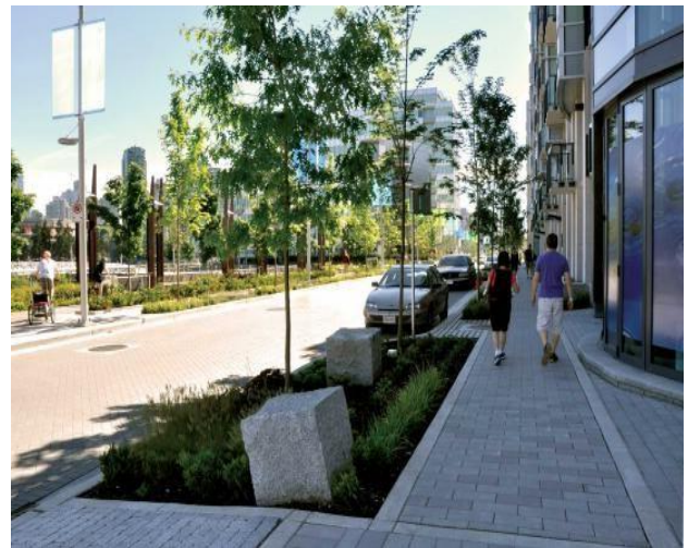
Figure 27: Permeable Pavers in Athletes Way at Columbia - Olympic Village
