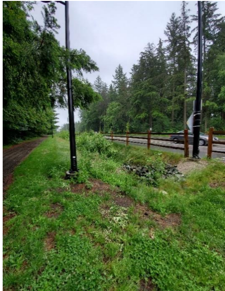
Figure 15: 100 Ave, Surrey, roadside bioswale
