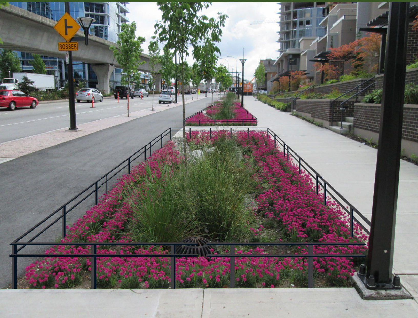
Rainwater Management Amenity at Lougheed Highway, Brentwood Town Centre, Source: City of Burnaby Town Center Standards
