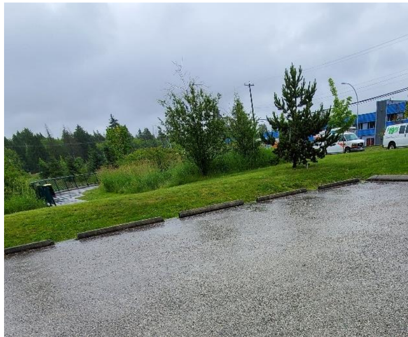
Figure 29: Sullivan Park Parking Lot Porous Pavement
