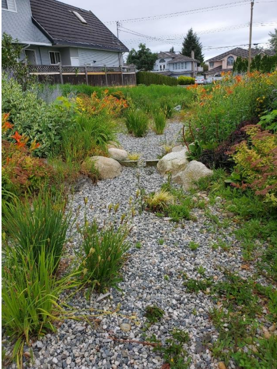
Figure 22: McCloskey – BC Hydro Rain Garden in North Delta
