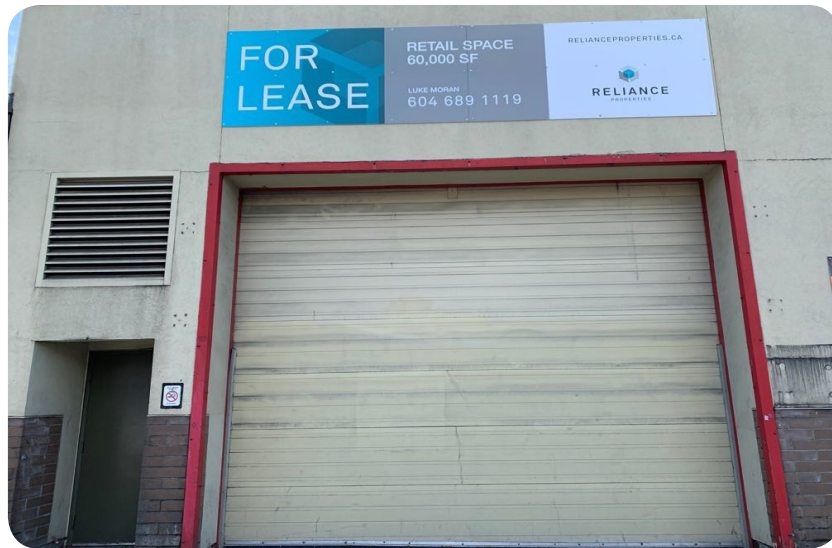
Figure 21. Undefined Infrastructure Source: Taken July 6, 2020
