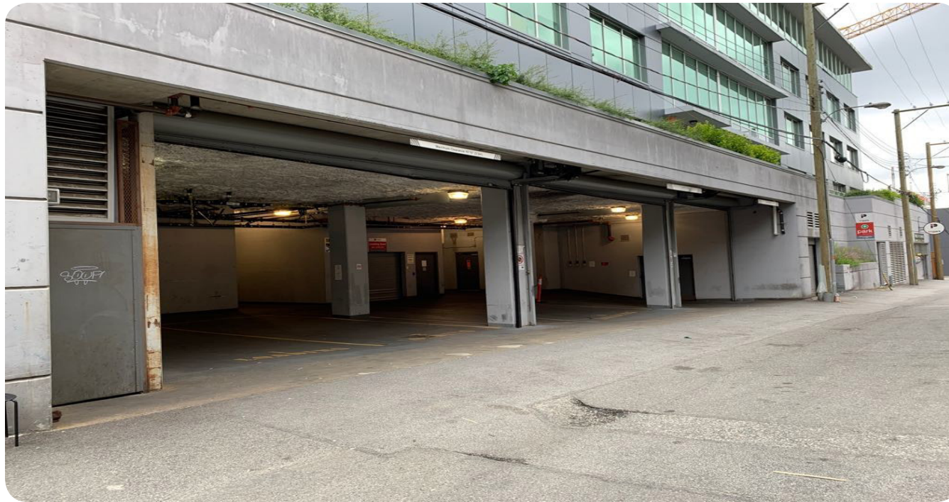
Figure 32. A Loading Bay Located Behind a Laneway Source: Taken June 30, 2020
