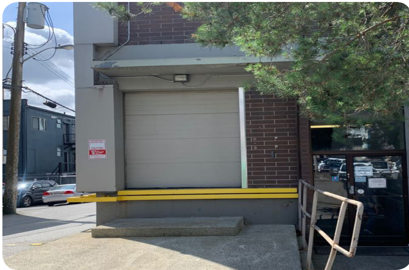
Figure 19. Exterior Loading Dock Source: Taken July 8, 2020
