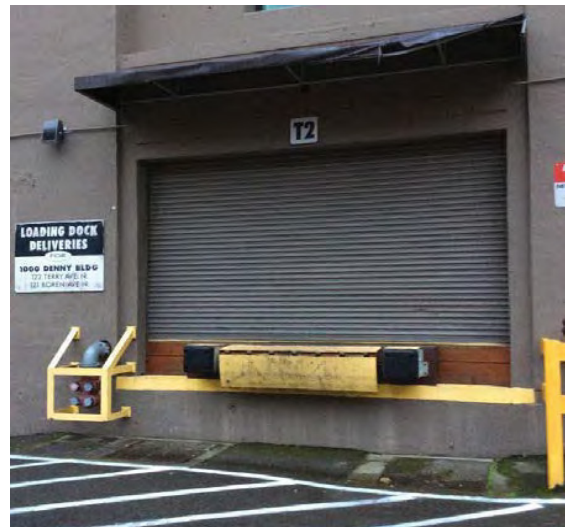
Figure 3-3. Closed Loading Dock
