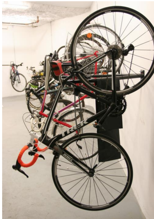
Figure 20. EOT secure bicycle storage (Onni Group in downtown Vancouver). 45
