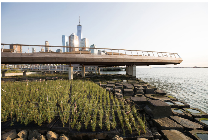
Figure 24: Tide deck during low tide, Hudson River PK, (n.d.).
