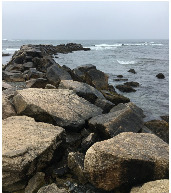
Figure 15: Rock groin - hard shoreline approach, photograph by Bob Bowie, (2019).
