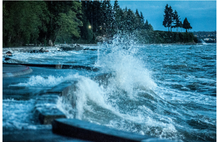
Figure 11: Waves hitting the seawall, photograph by Colin Knowles, (2013).
