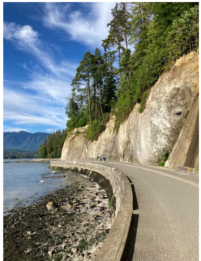
Figure 49: Existing site conditions
