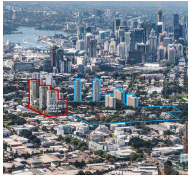
Figure 28: Waterloo Metro Quarter Post-Development. 278
