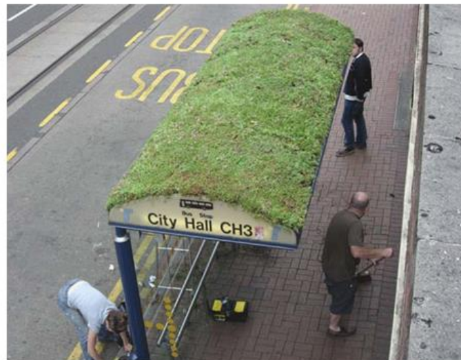
Image 11: Green roof: NACTO
