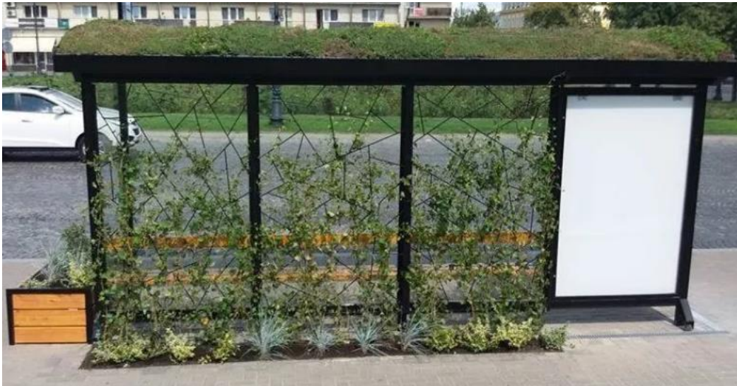
Image 12: Green roof: NACTO
