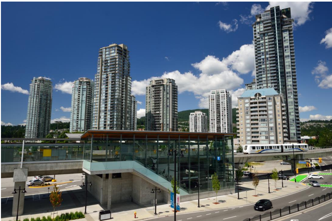
Figure 21. Lincoln station viewed from the southeast.
