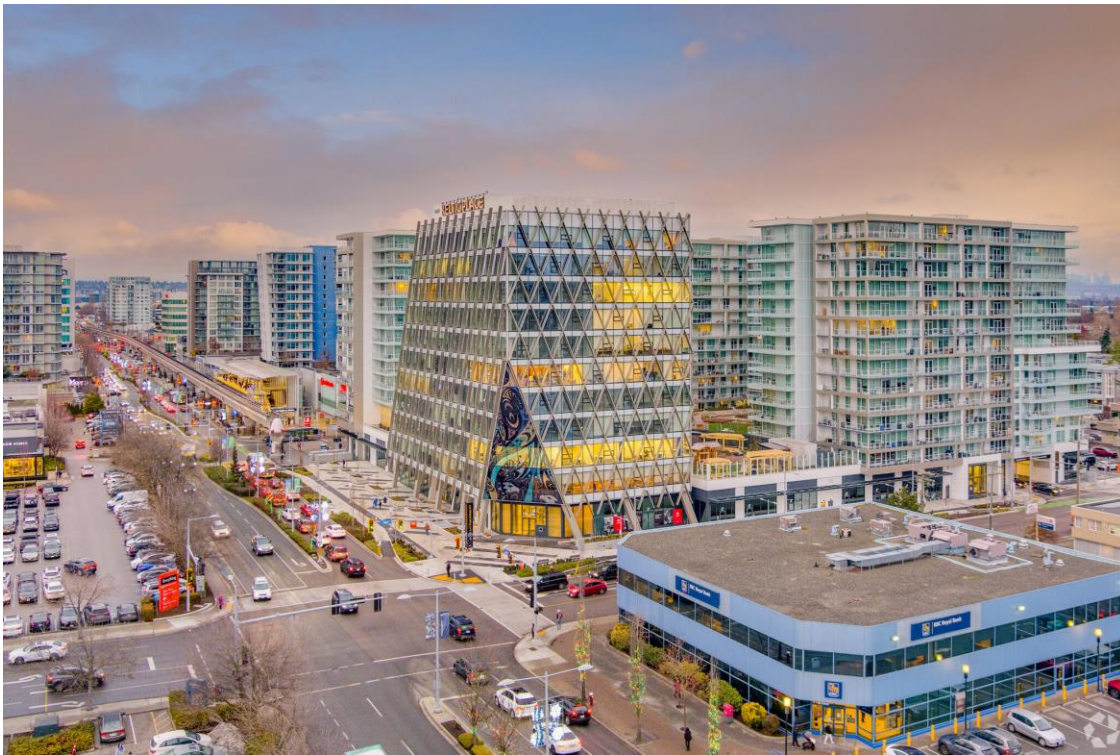
Figure 18. Streetscape at No. 3 Rd and Cook Rd near Richmond-Brighouse station.
