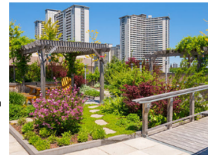
Intensive green roof on Hugh Garner Co-op (Toronto, Ontario)
