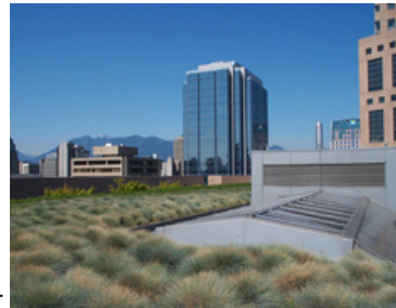
Extensive green roof on the Vancouver Public Library (Main Branch) (image credit: Terri Meyer Boake).
