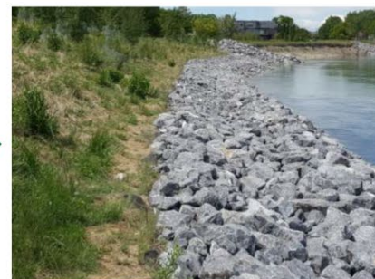
PICTURE 2 Site 4 in 2023, following works.
