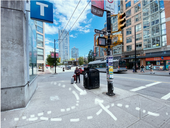
Figure 1. Significant sloped grading
