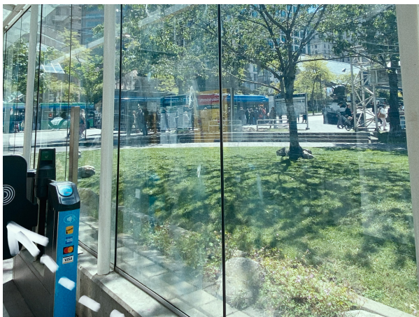
Figure 3. Clear glass barrier
