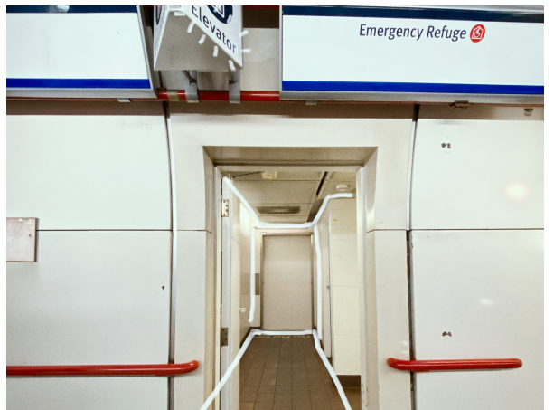
Figure 4. Corridor towards elevator
