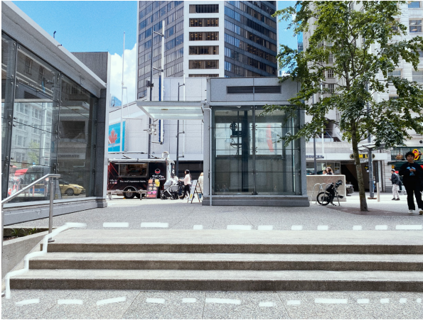
Figure 1. Short, wide, unavoidable stair
