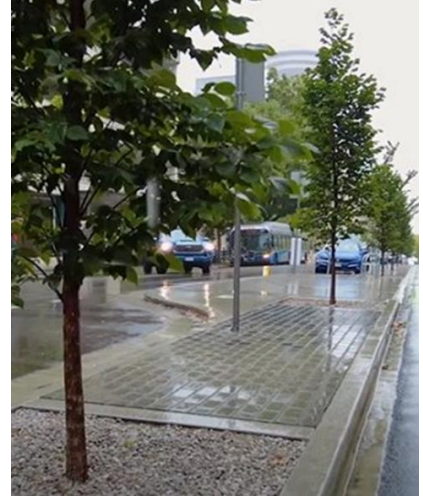
Figure 1-3 Green Rainwater Infrastructure - Permeable Pavement
