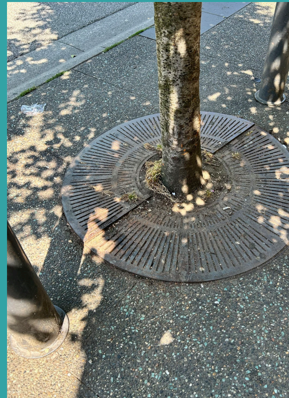
A tree in an upheaved tree grate. Photo taken in Granville Street, downtown.
