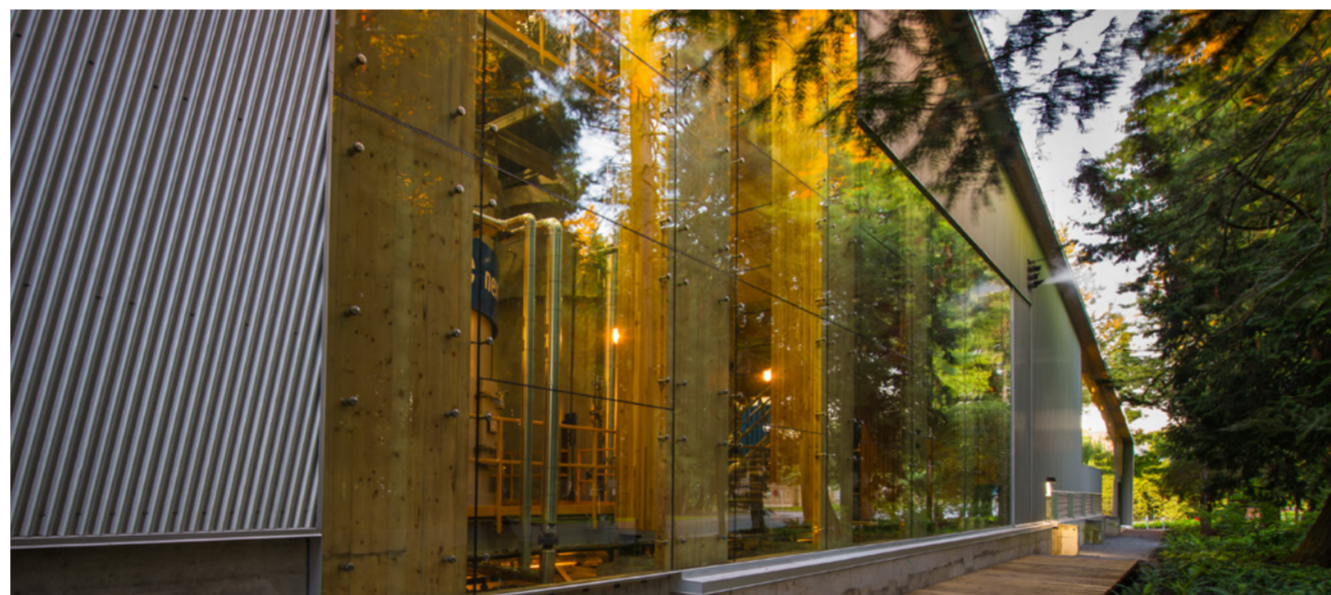
Glass wall on south side of the building
