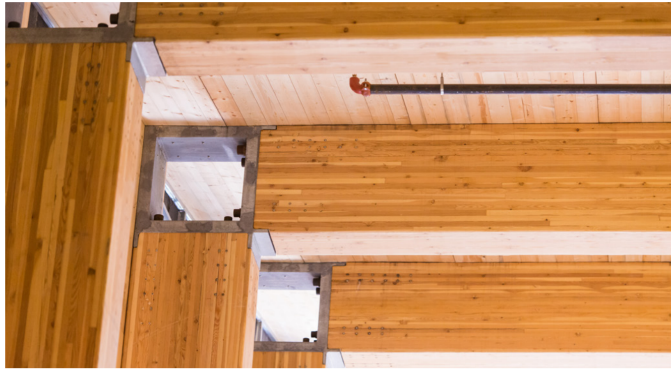
Glulam columns and beams with box connectors, and CLT roof
