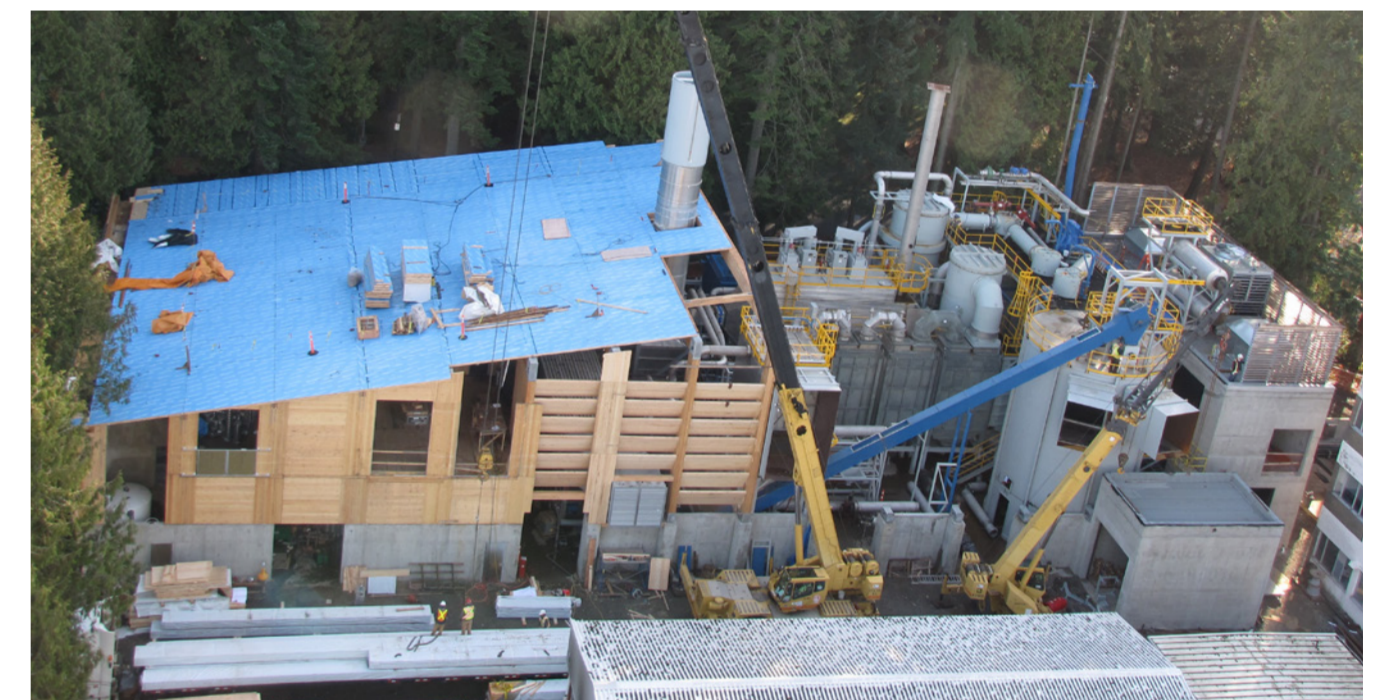
Building construction and equipment installation
