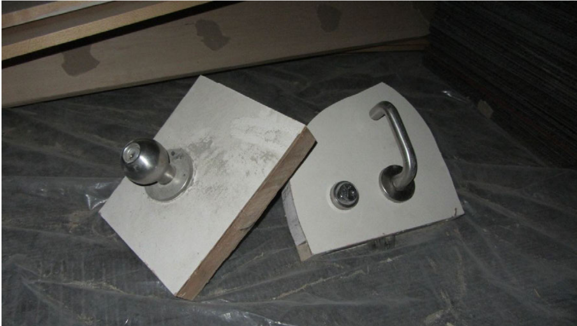
Figure 1 Door knob and door handle stored onsite for reuse in other UBC projects, The contractor mentioned that UBC favors keeping these door handles, Project: University Centre - Contractor: Scott Special Projects
