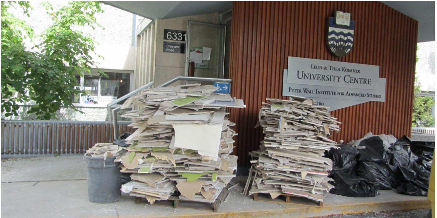
Figure 11 Drywalls, separated for recycling, Project: University Centre - Contractor: Scott Special Projects
