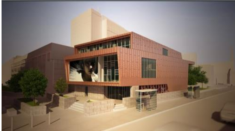
Figure 1 – The House Opened in 2014 – BREEAM Excellent standard
