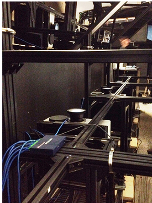
Figure 4: Photo of the hardware behind the IMW
