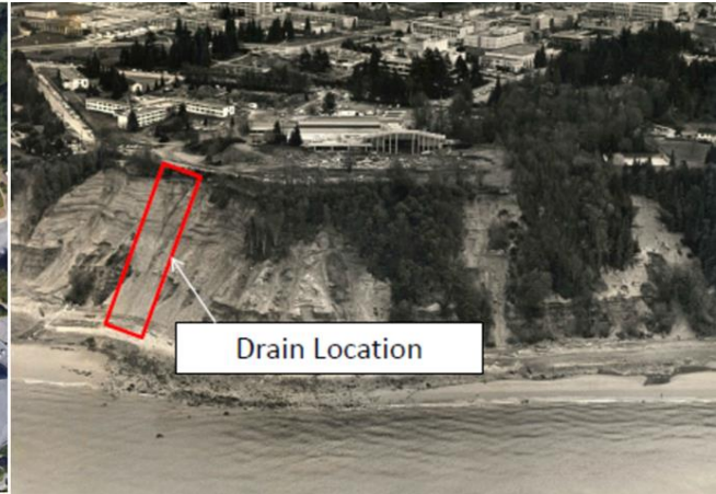
Figure 2 View of Spiral Drain from Cliff-side
