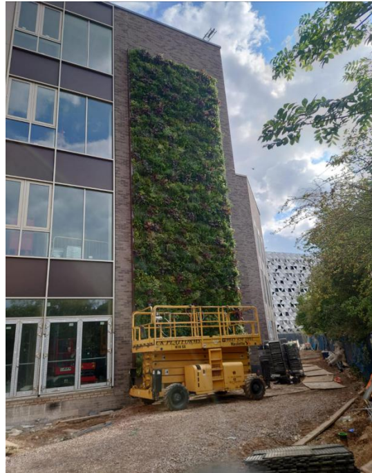
Figure 11. The exterior living wall on the UoL teaching and living center, Leicester, UK.
