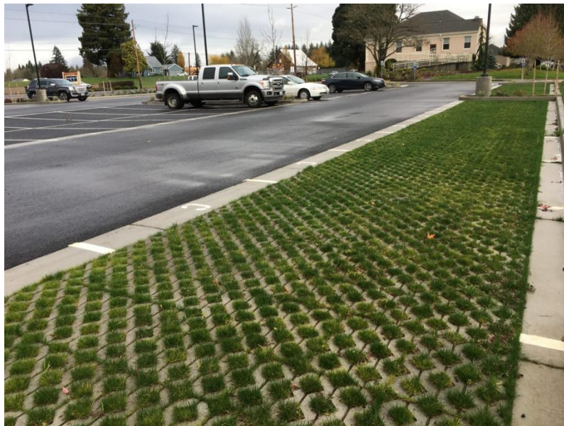
Figure 4. The lush appearance after the completion of paving turf stone pavement in the parking lot of Heritage Farm, Vancouver, WA.
