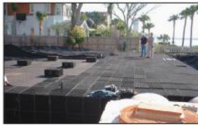
Installation of the Matrix® tank modules
