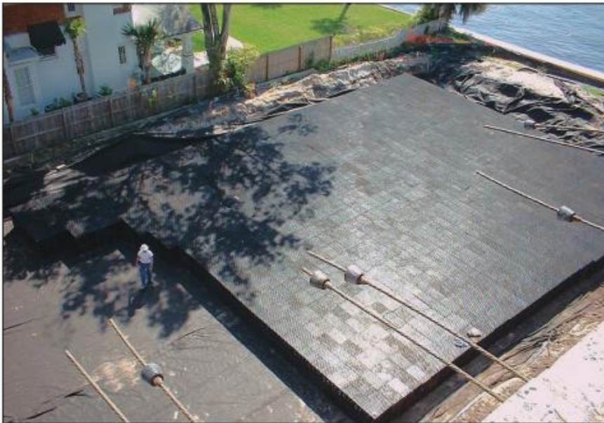
Installation of the Matrix® tank modules
