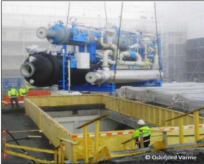
Figure 8: Unitop 43/28 BPY heat pumps from Friotherm during installation
