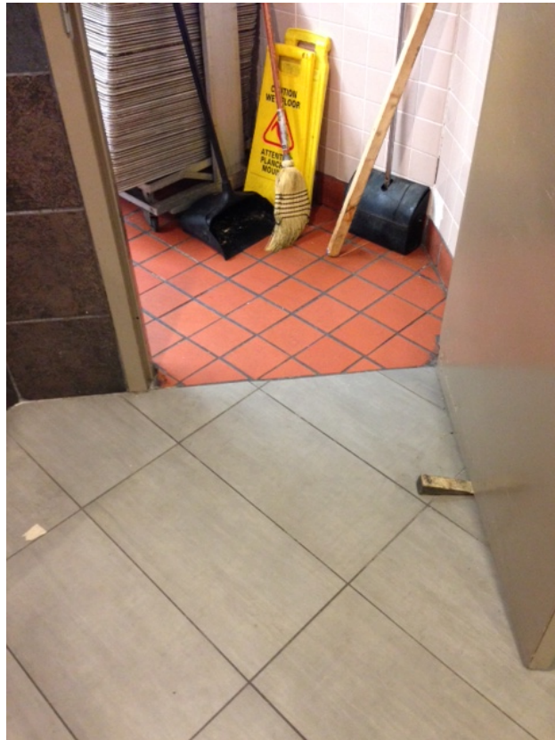
FIGURE 1: PVC tiles used in main cafeteria area, and the ceramic tiles required for the preparation area. (Photo by Ben Mattison)
