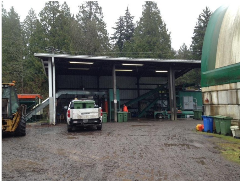
FIGURE 4 DOCKING STATION AT THE COMPOSTING FACILITY
