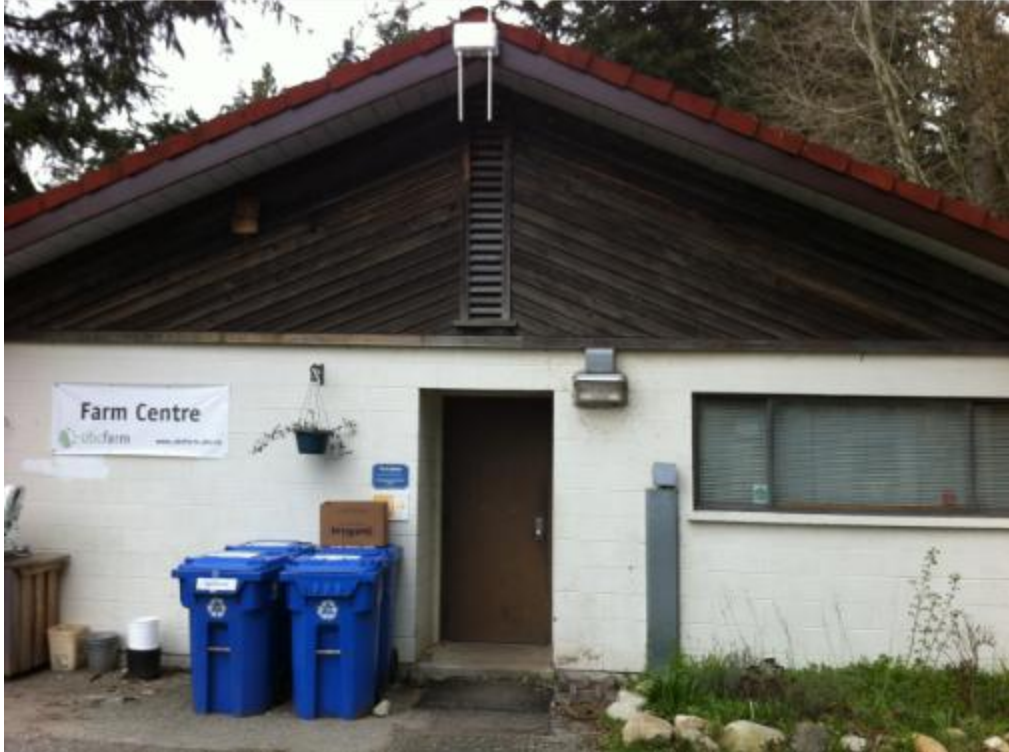
Figure 5.4 – Farm Center at the UBC Farm. Approximate roof area is 216m 2
