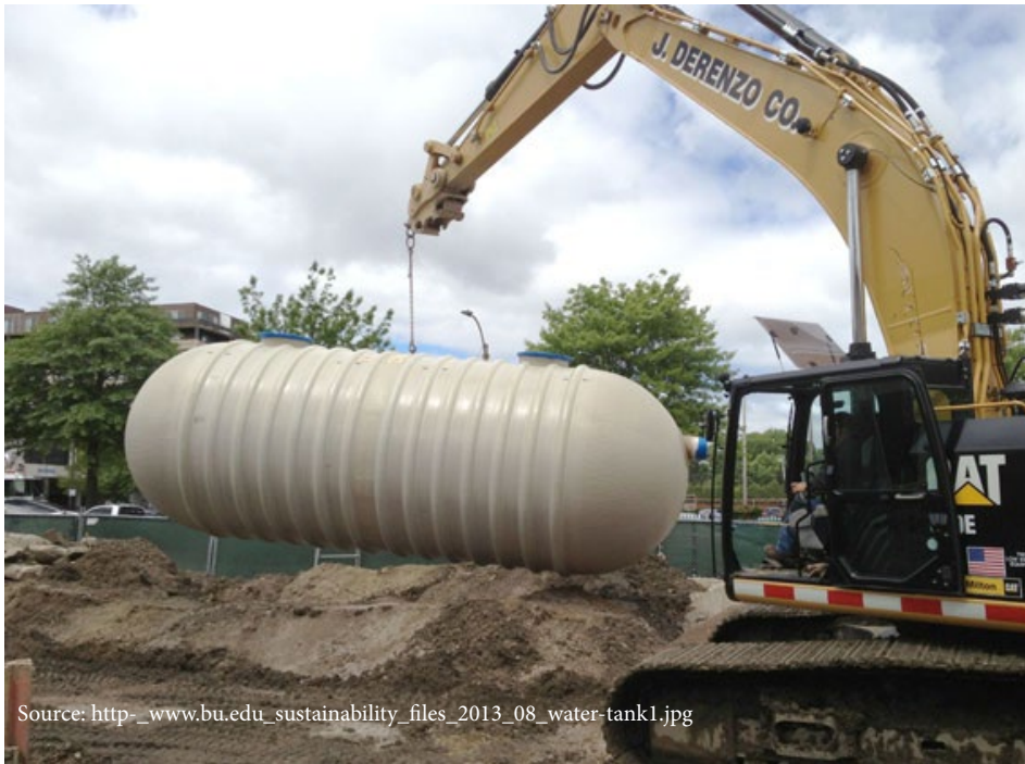
Figure 24. 15,000 gallon tank being installed at the New Balance Field on The University of Boston Campus.
