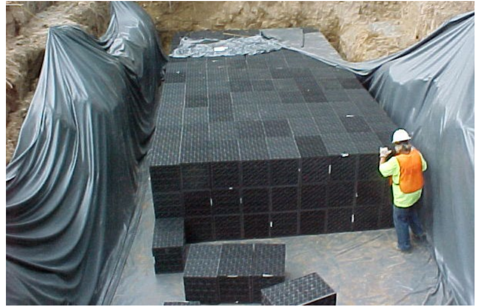
Figure 32. Installation of Rain Tank Modules
