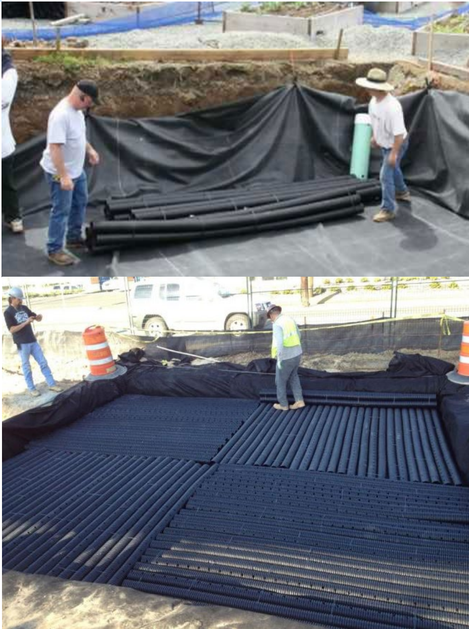
Figure 34. Installation of Storm Water Retention Chamber.
