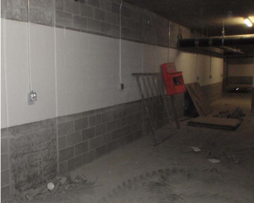
Figure 1 - P2 Parking Area Rough In for Seven EV Charging Circuits
