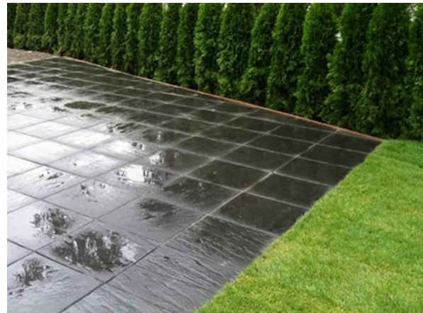
Figure 23: Concrete paving stones
