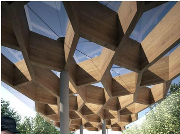
Figure 22: Laminated glass roof and honeycomb support
