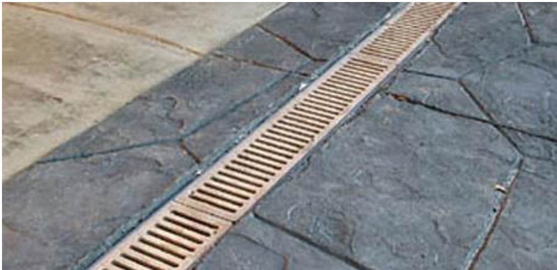
Figure 6: Typical channel drain
