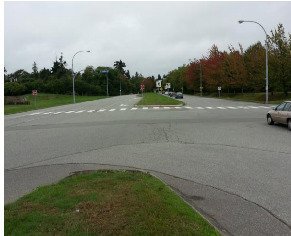
Figure 9. Photo of SW Marine Drive Crosswalk at Stadium Road
