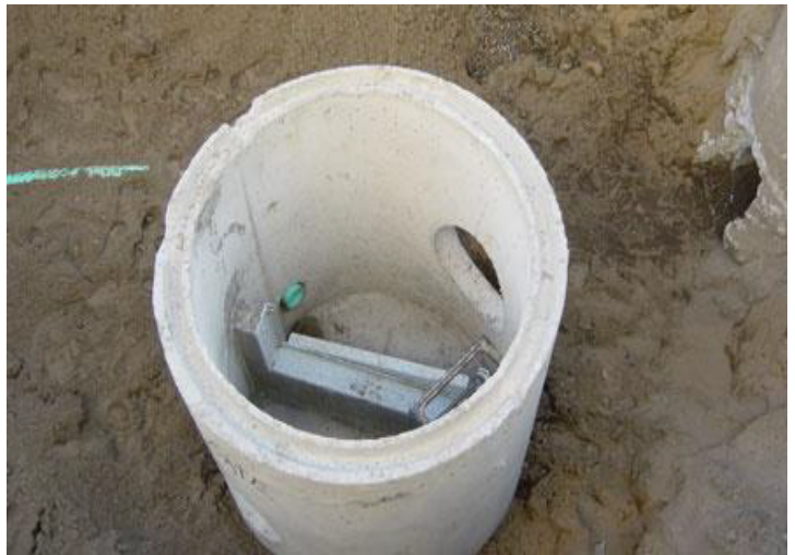
FIGURE 3 - STORMGATE™ FLOW MANAGEMENT CONTROL DEVICE WITH ADJUSTABLE WEIR (CONTECH ENGINEERED SOLUTIONS, 2014)
