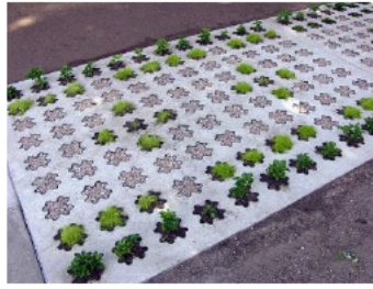
Figure 11: Interlocking concrete pavement (Green Innovations, 2010)
