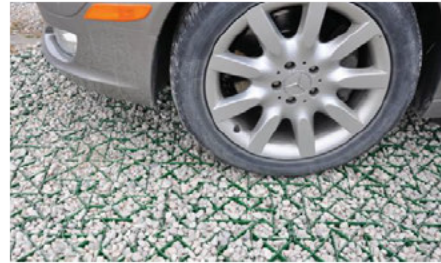
Figure 12: Permeable pavement system (Green Innovations, 2010)
