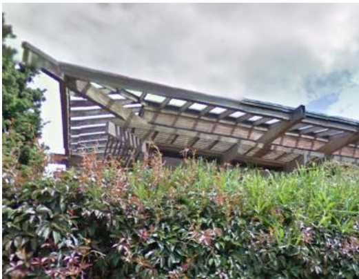
Figure 2: Joists and Skylights Seen in Existing Garden Pavilion
