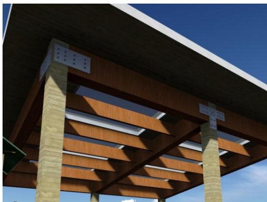
Figure 4: Oversized Joists Support Skylight Panel
