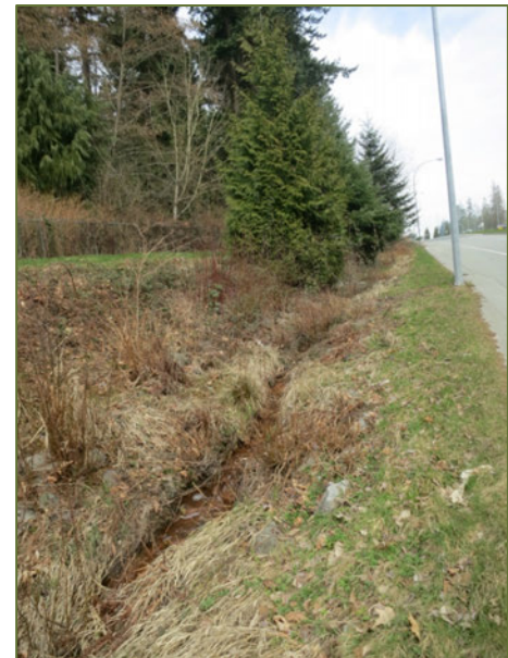
Figure 9: 16th Ave Drainage
