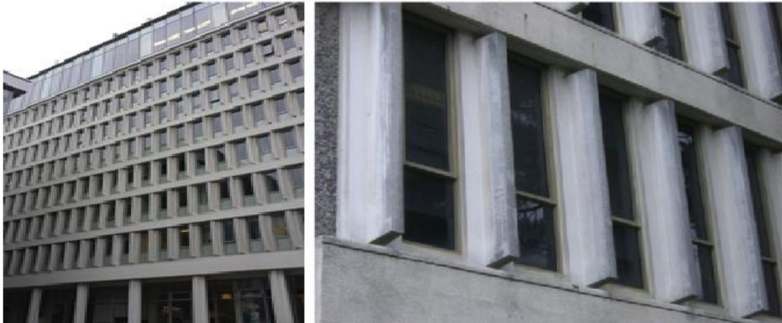
Figure 3 - Precast exterior wall on west
