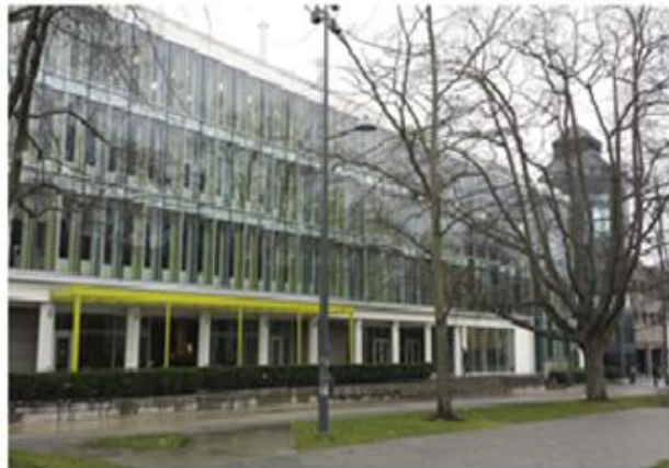
Figure 8 - Building after second Renovation
