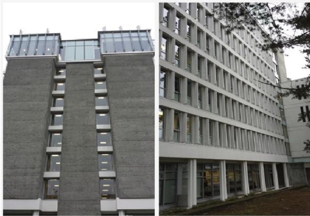
Figure 4 - Office Block Southwest
