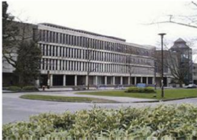
Figure 7 - Building before Renovation
