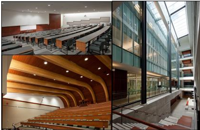
Figure 9 - Interior renewal and expansion
