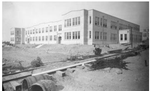
Figure 1 Construction of the "temporary" Geography Building circa 1925. ©UBC
