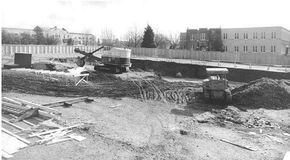
Figure 3. Lasserre Ground Work 7
