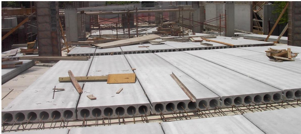
Figure 8. Hollow-Core Concrete Flooring 21
