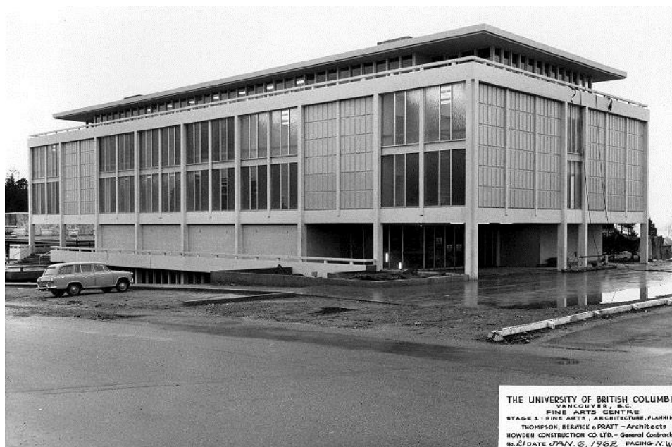
Figure 6. Lasserre Finished Construction 10
