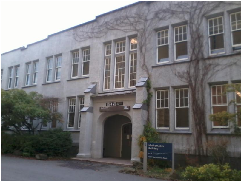
Figure 1. Front entrance of Math building.
